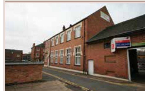
Re-purchase of the former parish hall as part of a larger building project at the church
