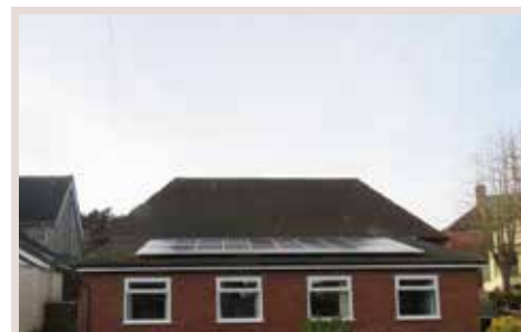
Solar panels installed
